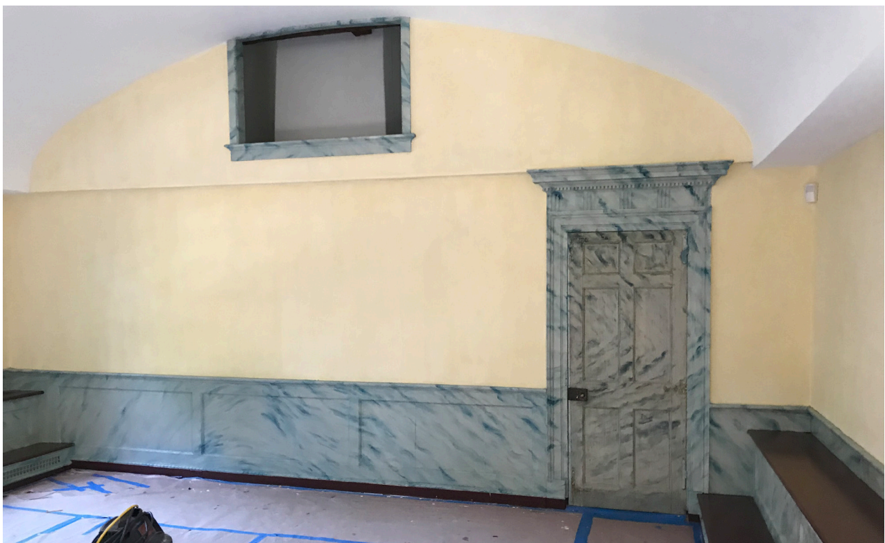
After wall and woodwork treatment
