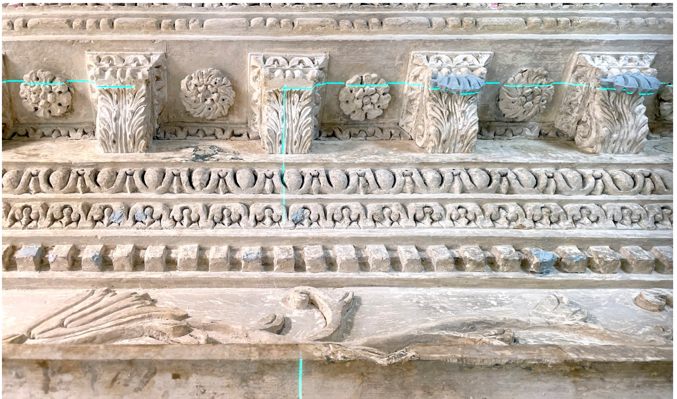
During repair and element replacement
