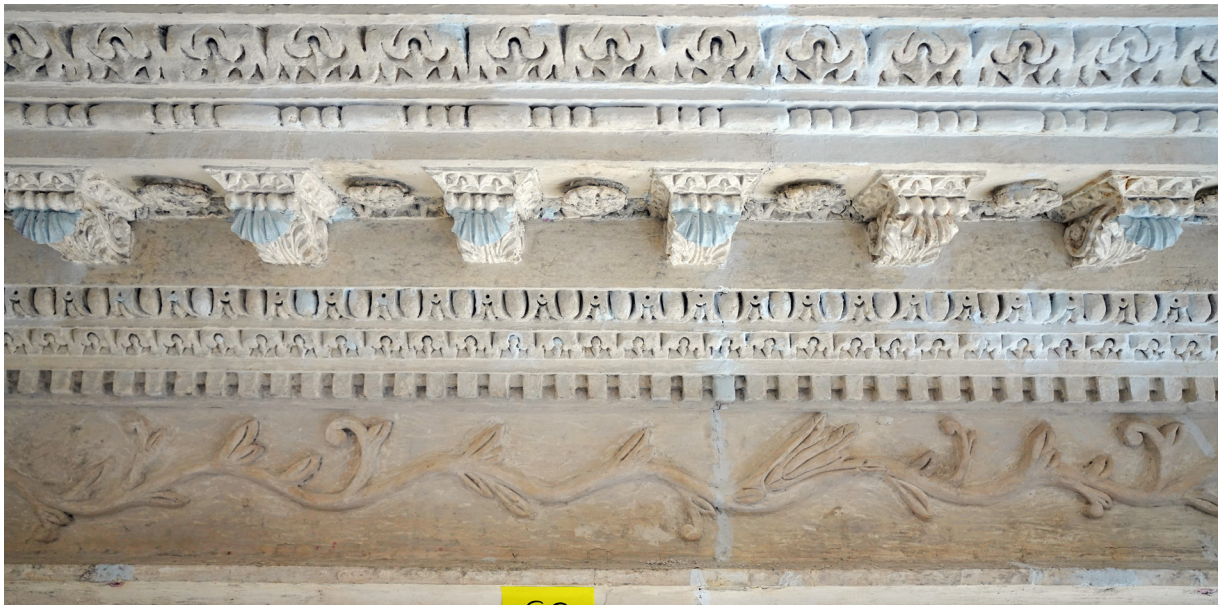
After paint removal and repair
