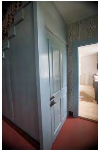
Stair Passage after treatment
