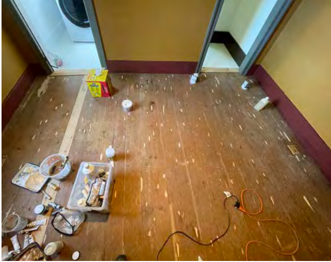
Laundry Room floor during fill installation
