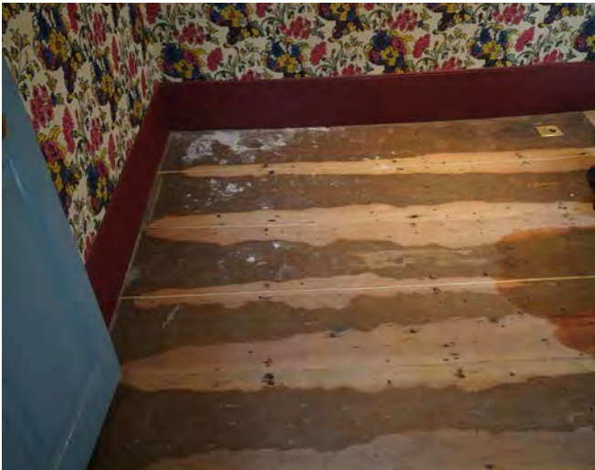
Parlor floor before treatment
