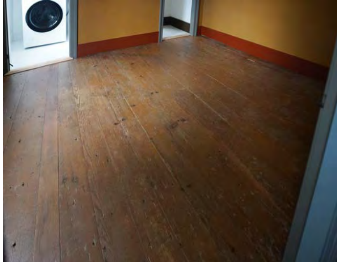
Laundry Room after treatment
