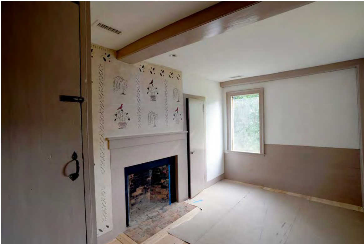
Kitchen Chamber after treatment
