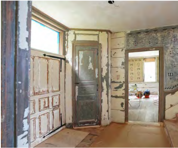
Stair Hall before treatment
