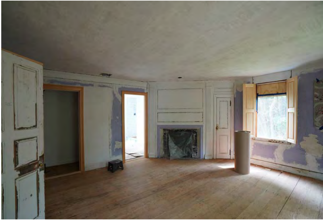
Parlor Chamber conditions before treatment
