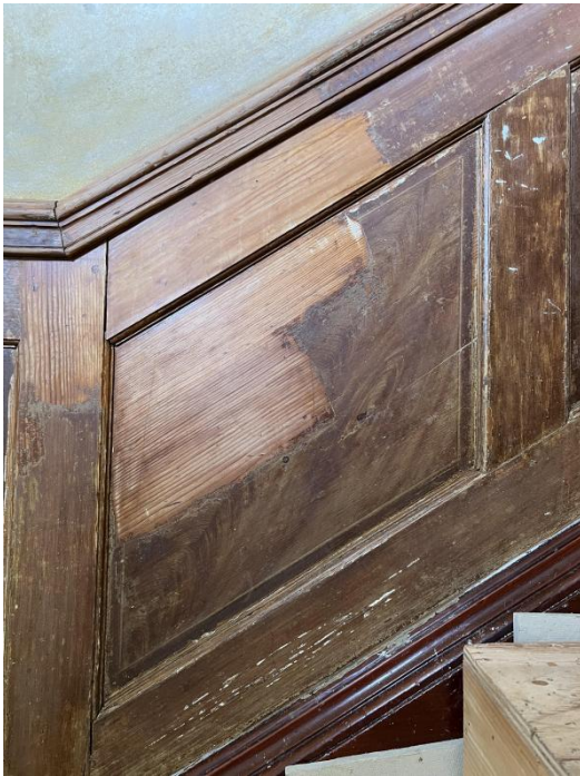
Image 22: Wainscoting with finishes partially burned off during the 1950s (Source: Kelsey Britt, 2022).
