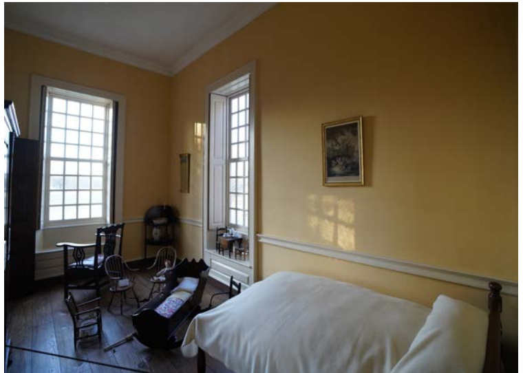
NW Bed Chamber after installation. Distemper walls, Linseed oil paint wooden elements, Limewash ceiling
