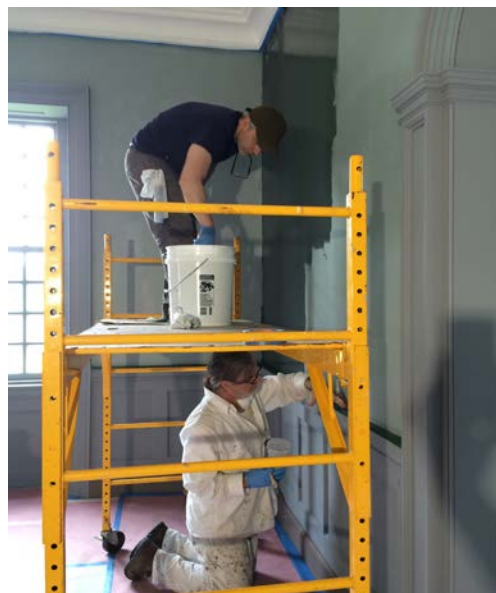
During installation of Verdigris paint on wooden elements and dark grey Distemper walls
