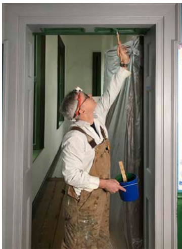
During installation of Verdigris oil paint
