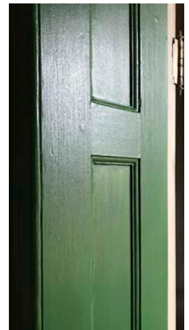
NW Bed Chamber after installation. Distemper walls, Linseed oil paint wooden elements, Limewash ceiling
