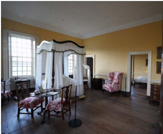
NW Bed Chamber after installation. Distemper walls, Linseed oil paint wooden elements, Limewash ceiling
