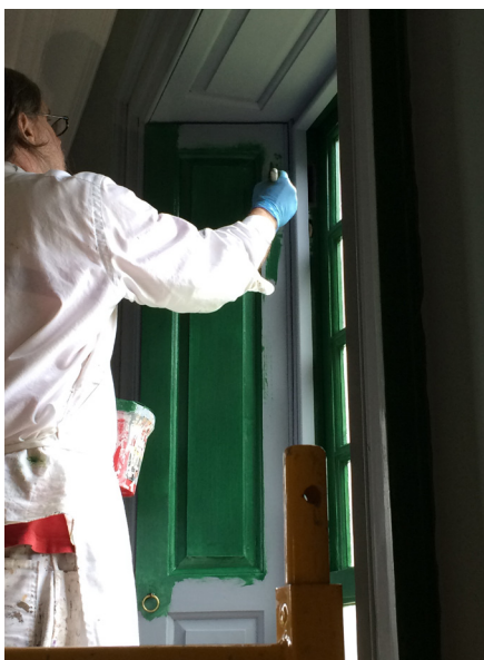
During installation of Verdigris paint on wooden elements and dark grey Distemper walls
