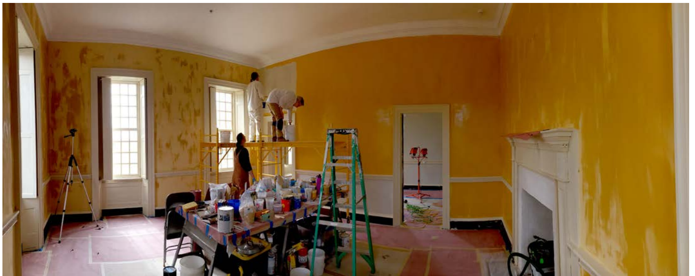
During installation of Distemper paint
