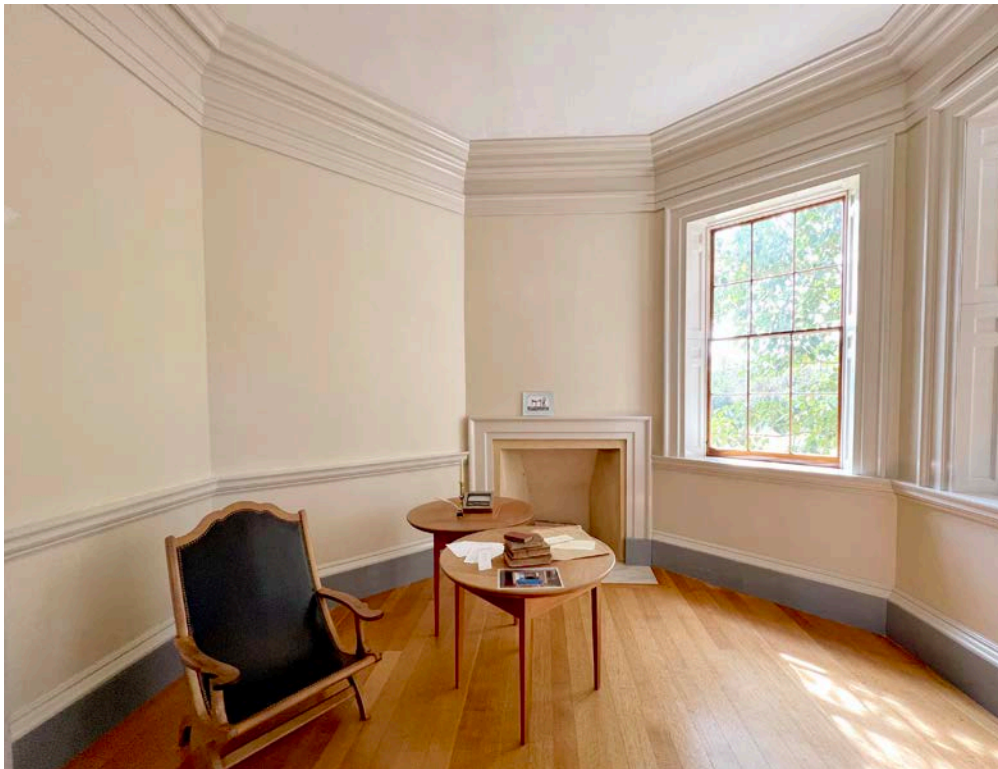
Bedchamber -Linseed oil satin walls and gloss oil woodwork, limewash ceiling
