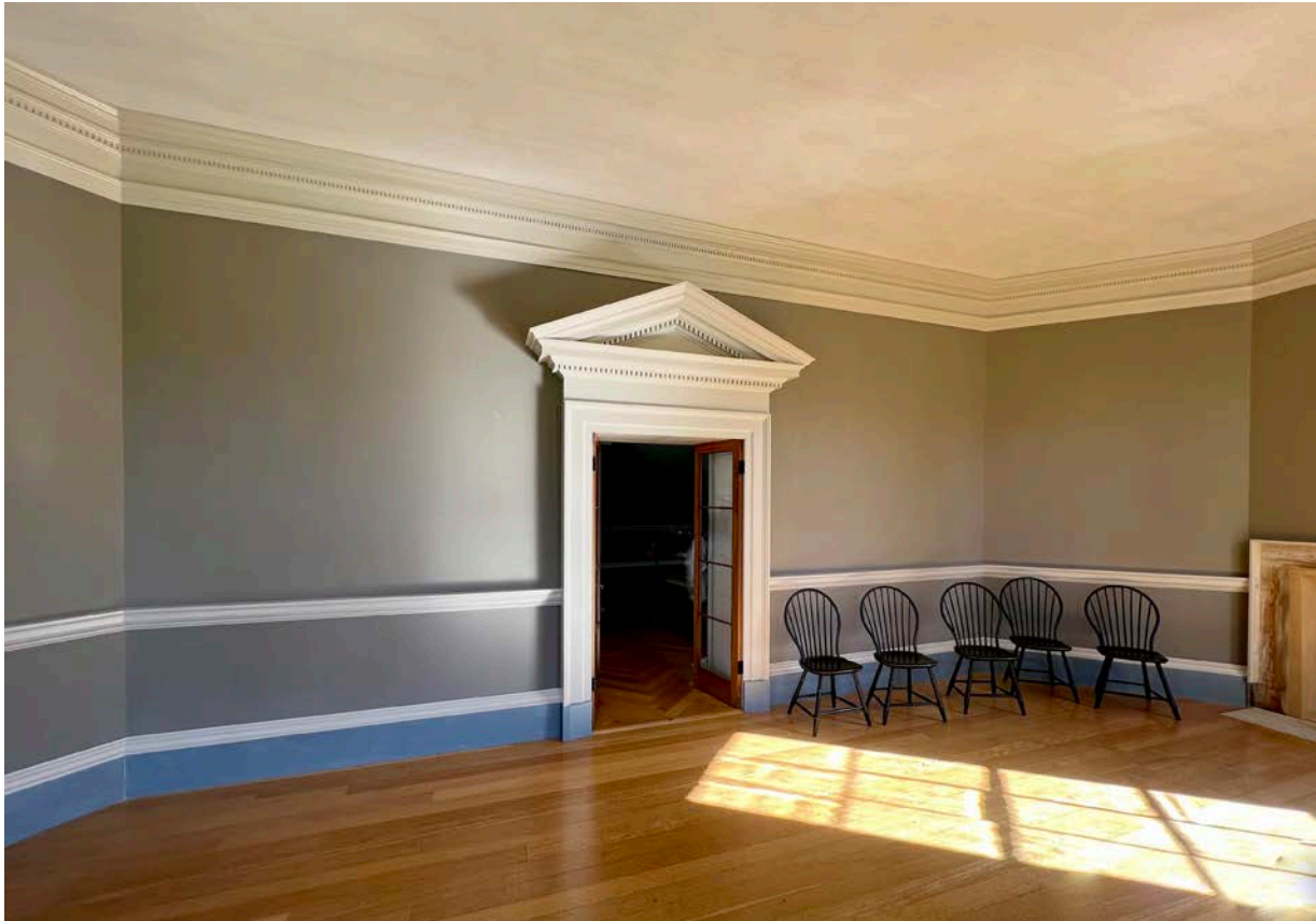
Parlor- Distemper walls and gloss woodwork, limewash ceiling
