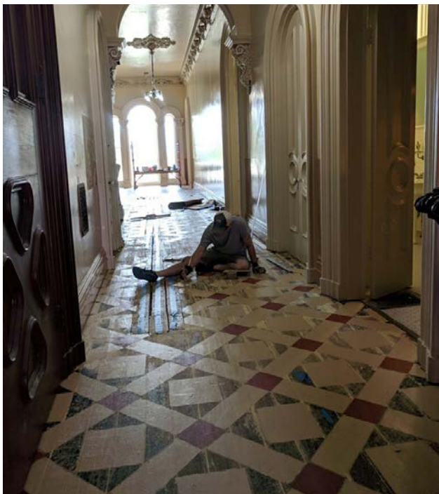
During floor restoration
