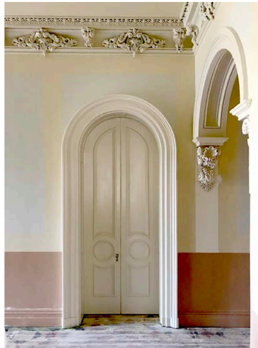
Hall walls and doors after treatment
