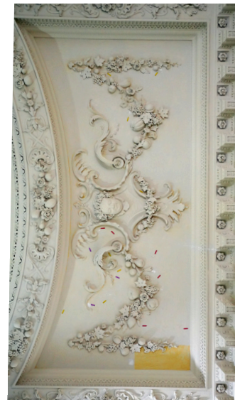
Casein paint removal/ plaster repair
